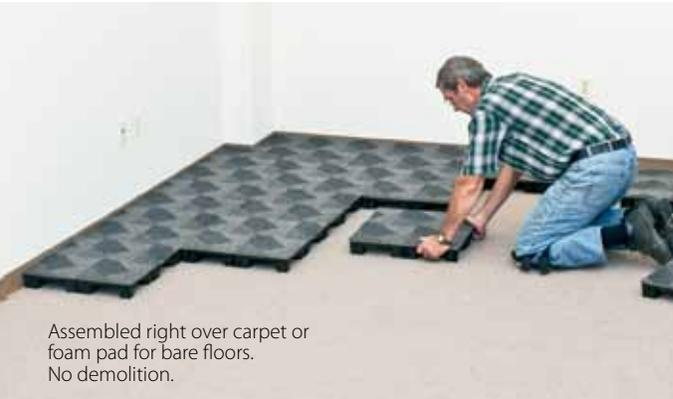
Assembled right over carpet or foam pad for bare floors. No demolition.
