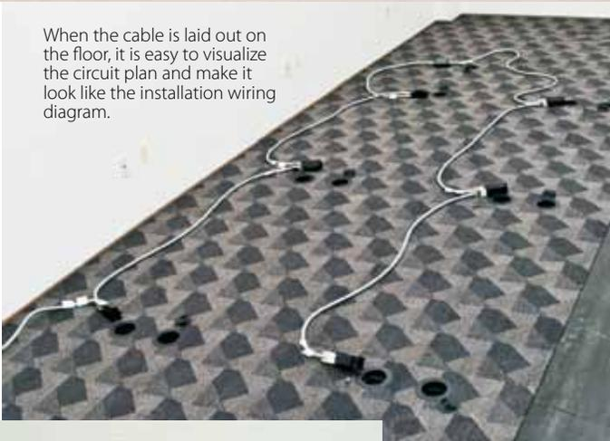
When the cable is laid out on the floor, it is easy to visualize the circuit plan and make it look like the installation wiring diagram.
