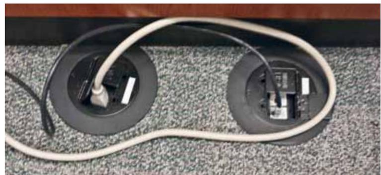
*Power and data outlets are universal and interchangeable with the ports in the floor. Locate power and data anywhere in the room. Move them anywhere in the room.*
