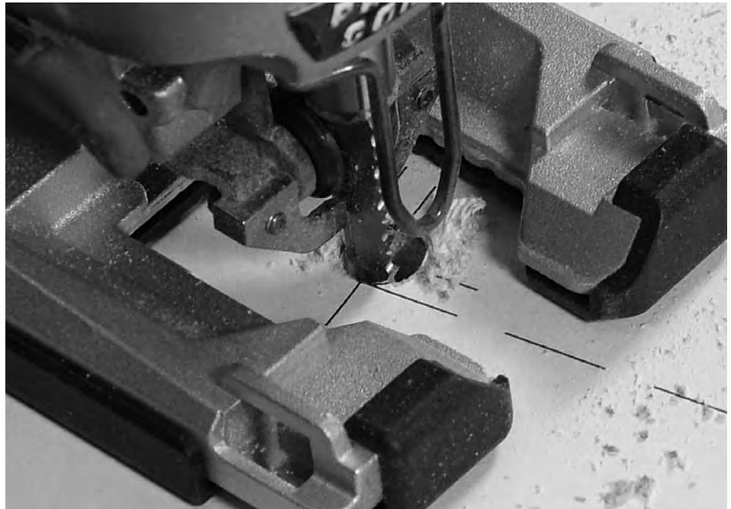
Place the jigsaw at the corner marking. Remove the layout line with the kerf of the saw cut for a factory fit. You must have the skill to saw a straight line within the tolerance of the width of the saw blade. Saw from corner hole to corner hole. Remove the remains of the paper template when this step is finished.
